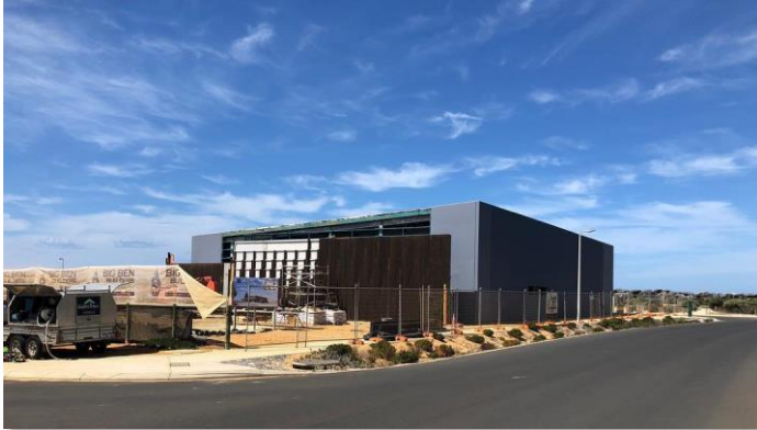
Construction progress – North Elevation
