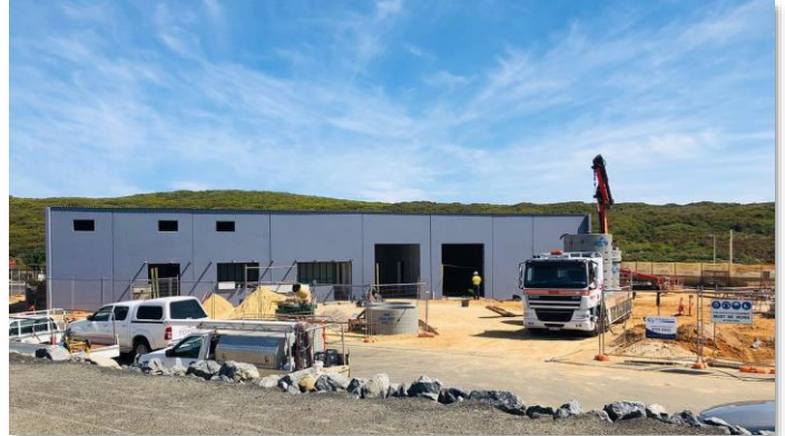
Construction progress – East Elevation
