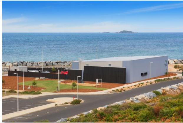
OGA's new processing facility with Flinders Bay Abalone Ranch in the background
